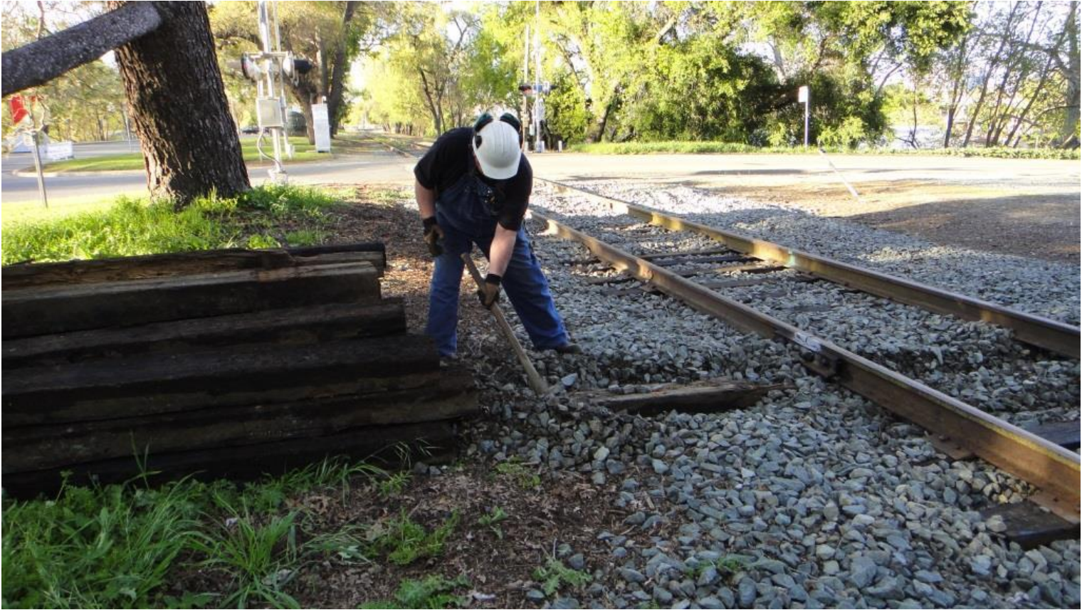
Harry digs out the remnants of a tie crushed by the Jackson 125 tie-exchanger
