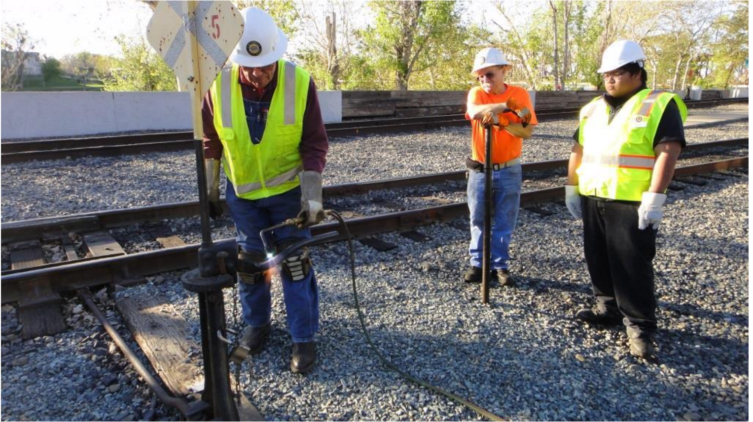
Cliff wielding his magic fire-stick to heat the misshaped switch handle so that Mike H. and Anthony could bend it straight
