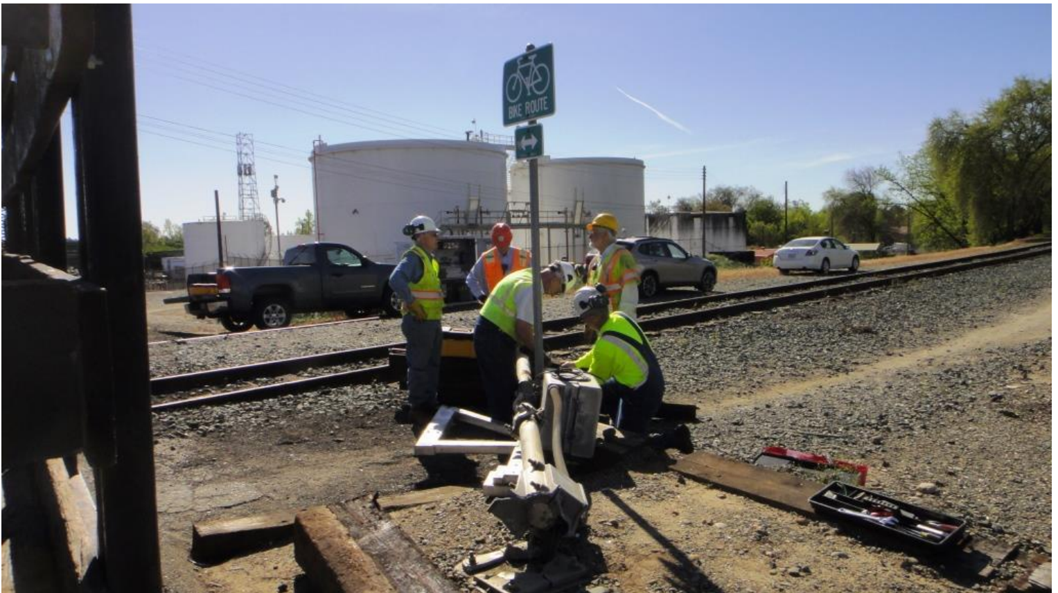
Clem and Dave Megeath prepare the mast for the big lift
