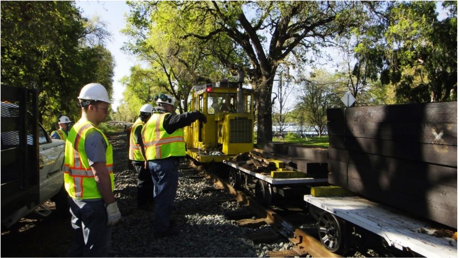
Meanwhile, back at the MOW work-site, Chris C. directs Mike F. in the Kalamazoo to the perfect stopping position
