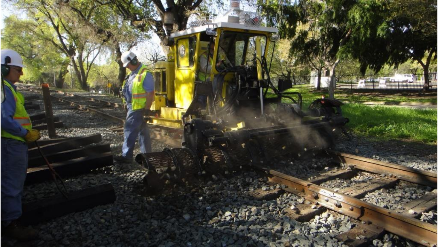
Alan brings the scarifier in to dig out new tie-cribs
