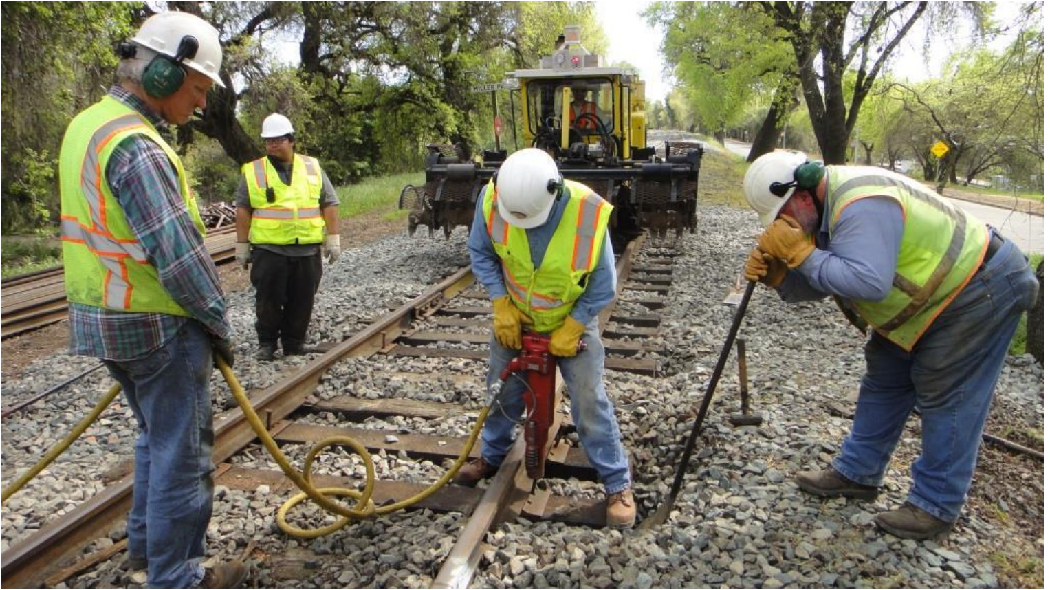
Mike W. dives the final spikes with Steve guiding the hose and Frank nipping the tie
