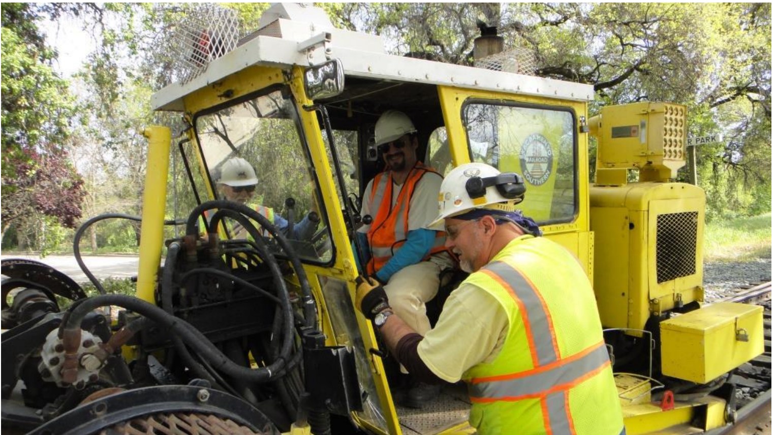
Meanwhile, Alan and Mike F. train Jose in the operation of the scarifier
