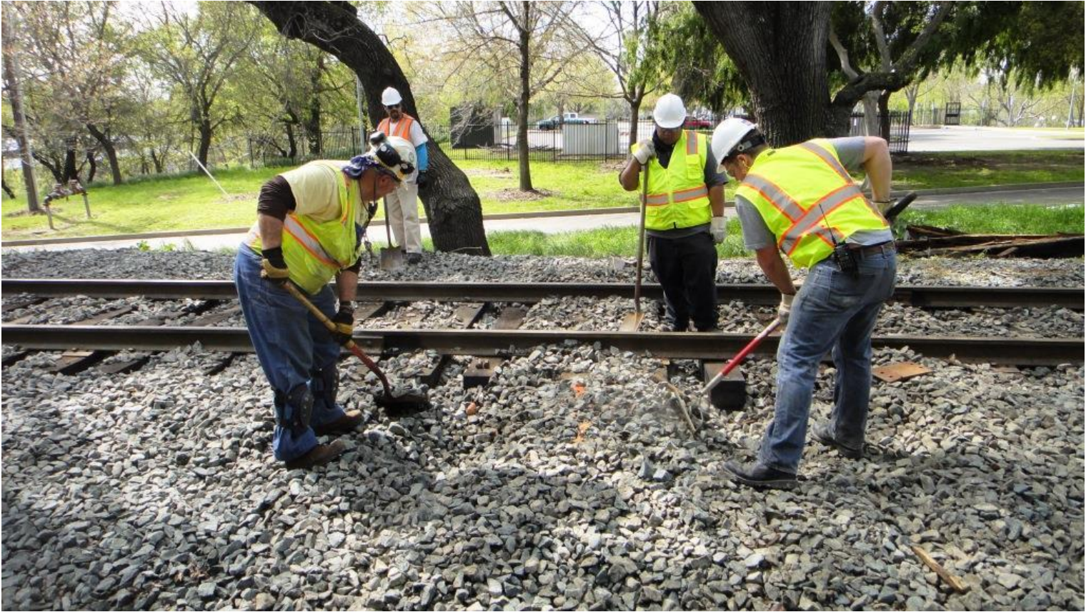
Jose, Mike F., Anthony, and Chris N. fill in the cribs around the new ties with plenty of rock for tamping
