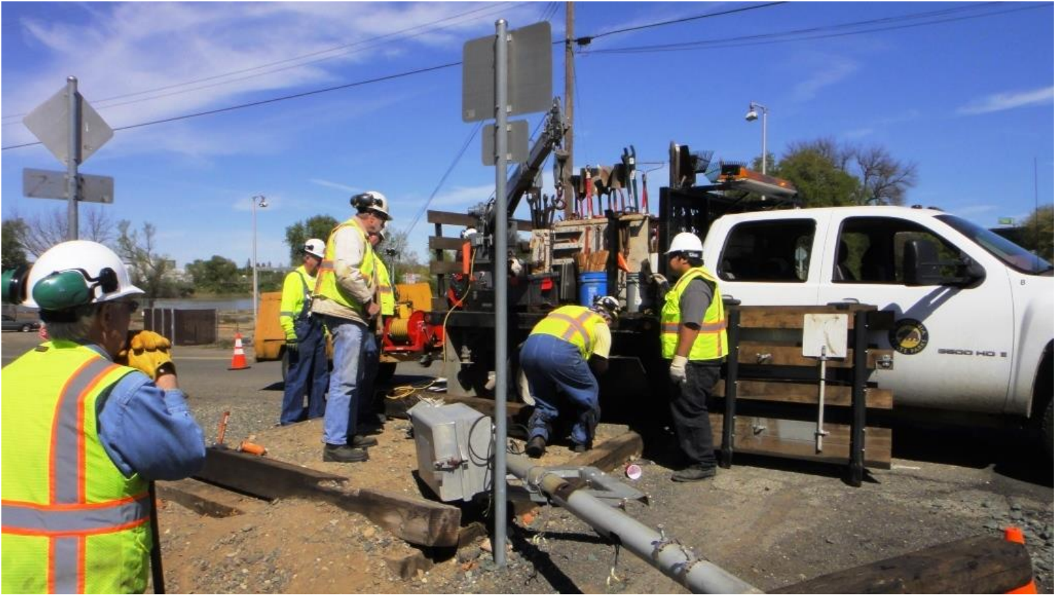
The crane on the MOW Team's trusty Chevy Truck is deployed
