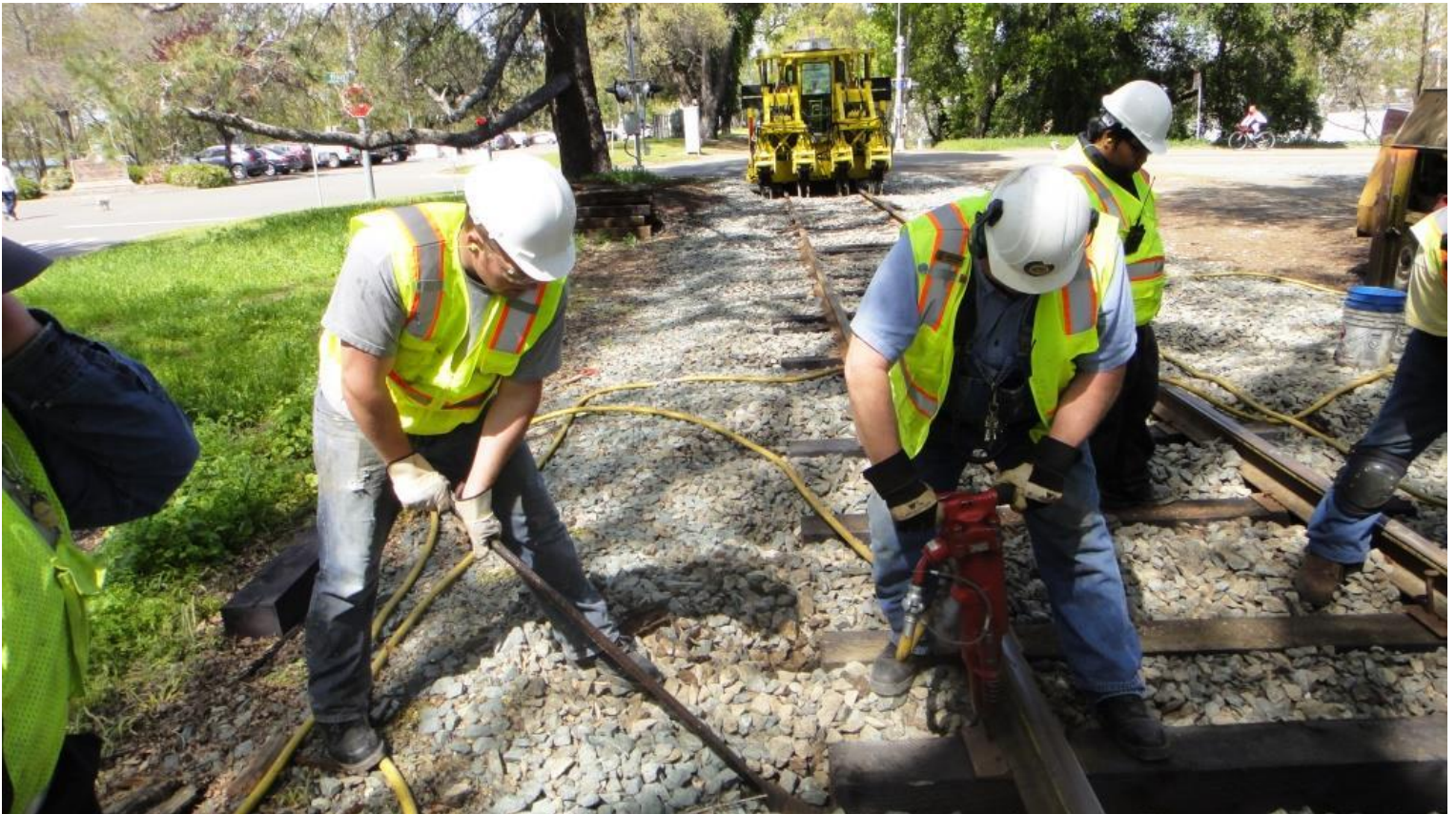
Chris N. nips-up the tie while Chris C. drives a spike with the pneumatic spike-driver
