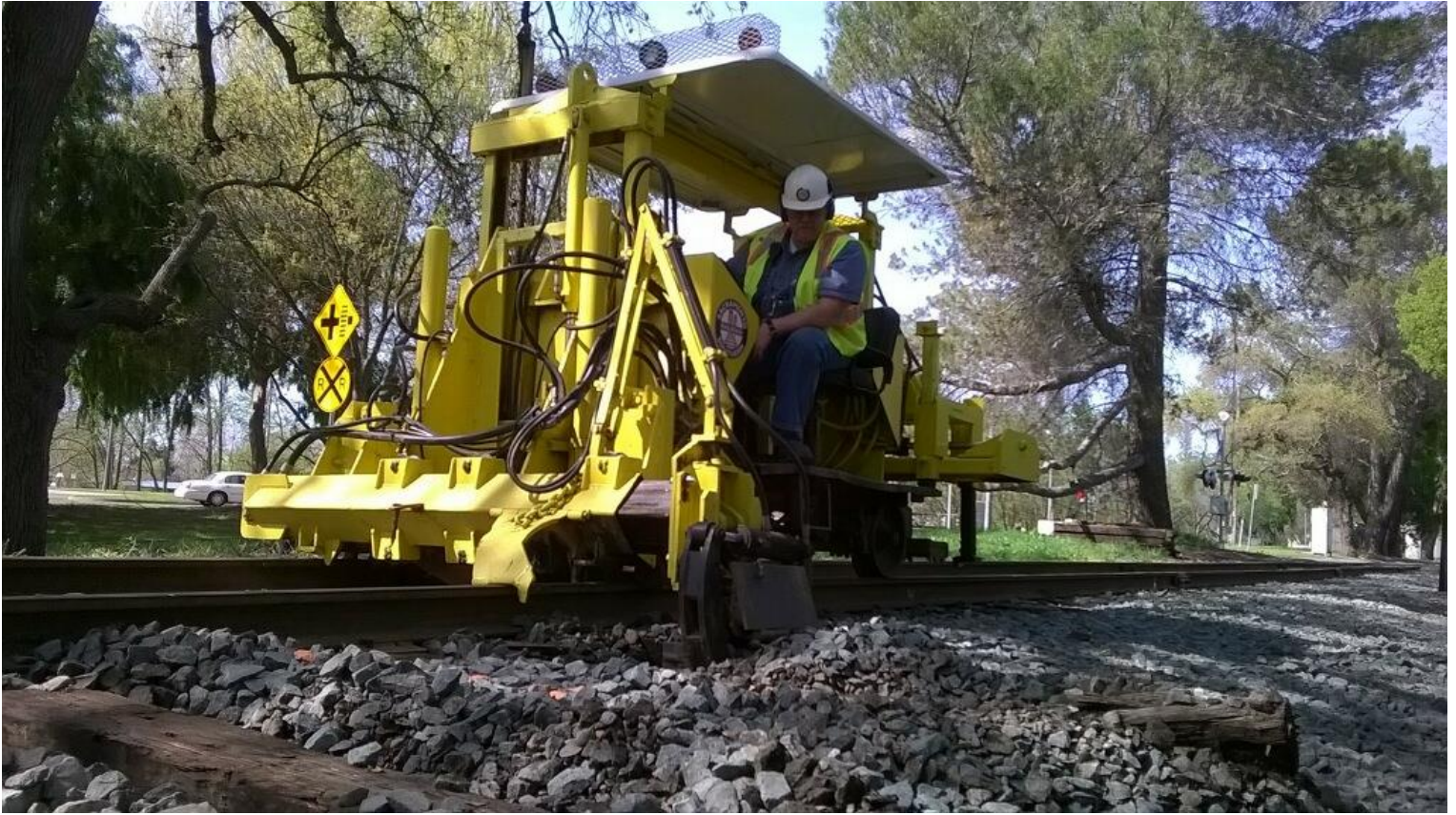
Chris C. on the Jackson 125, pulls a bad-tie out from under the rails
