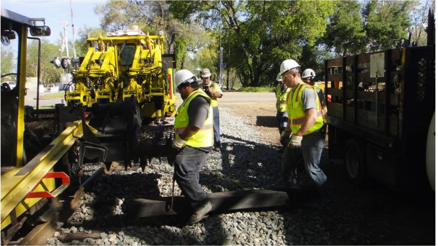
Anthony and Chris N. position another tie for installation
