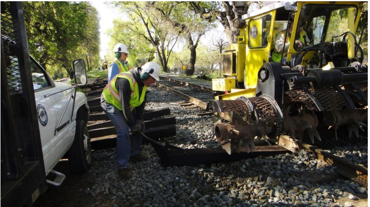
Steve guides a new tie into place
