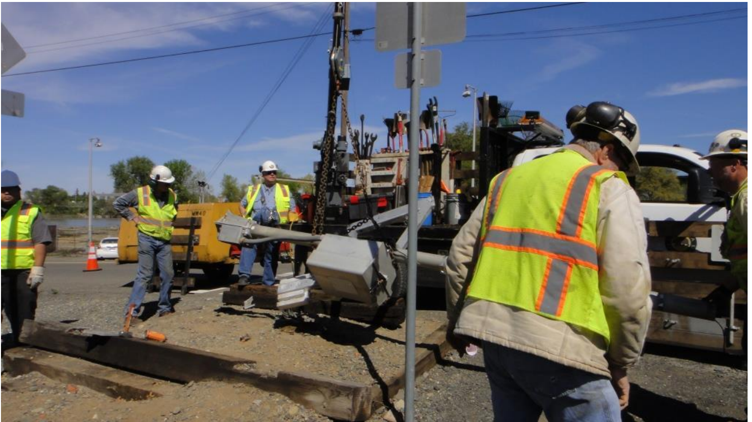
The signal mast is airborne! Chris C. controls the crane as Mike F. and Alan prepare to guide it into the Dodge
