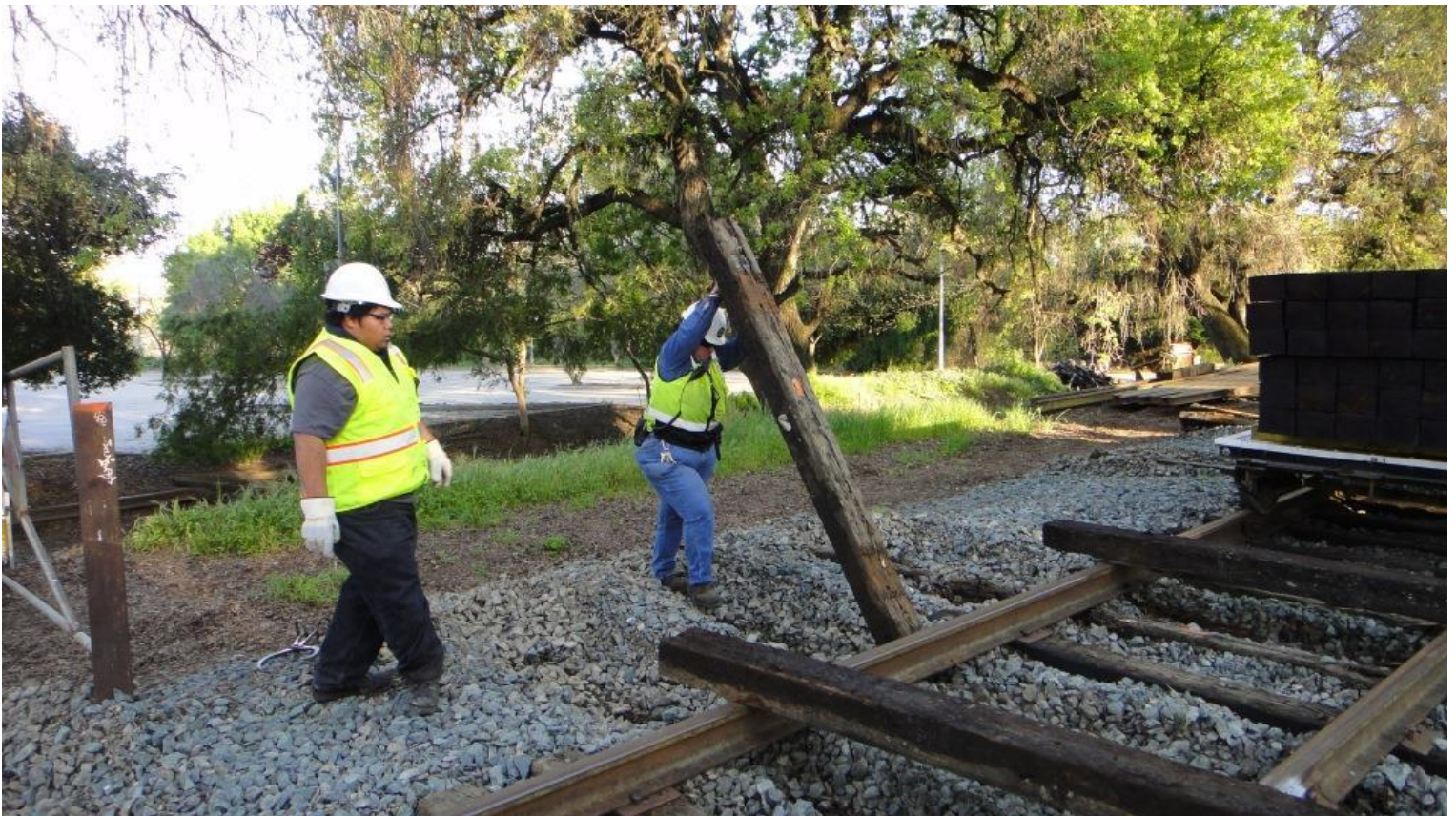
Heather tosses a tie onto the rail to be relocated to the dead-tie pile
